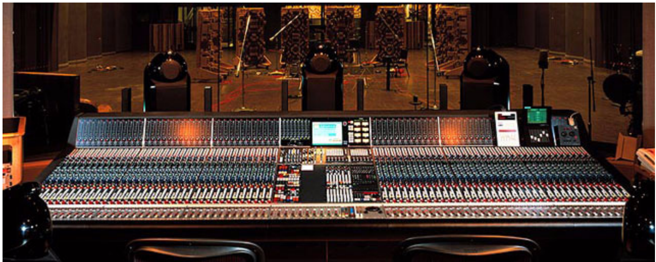
The Neve 88RS at Skywalker Sound in California
