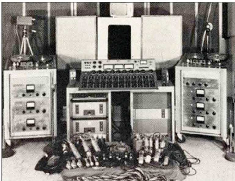
**Wally Heider's Remote Recording Rig, with 610 Console**
